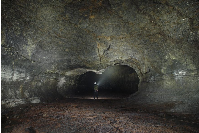
Fig. 2-25. Downward bulge in mid-ceiling. View is downstream. Longitudinal crack along middle of bulge is theorized to have formed as result of weight of the accreted lining (roof). See Fig. 2-8 and 2-9 for location (L15).
